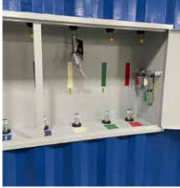
EXTERNAL HOSE REEL HOOKUP (IN PROGRESS INSTALLATION)
